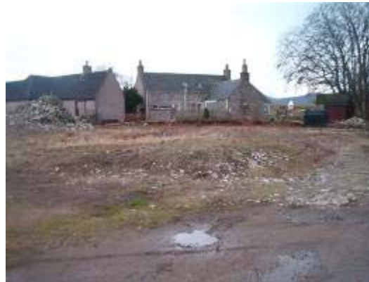
Fig. 5 : Proposed site as existing, post demolition work
