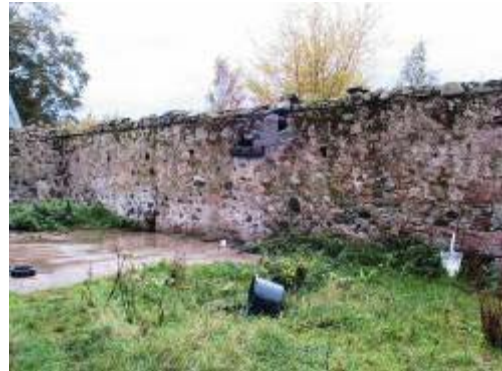
Fig. 4 : Ruins of former barn
