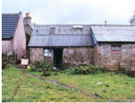
Fig. 2 : Partial exterior view of formerly existing steading
